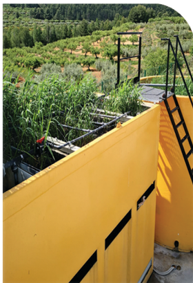
Modular METland® treating Wastewater (25m 3 /day , 200 pe)
